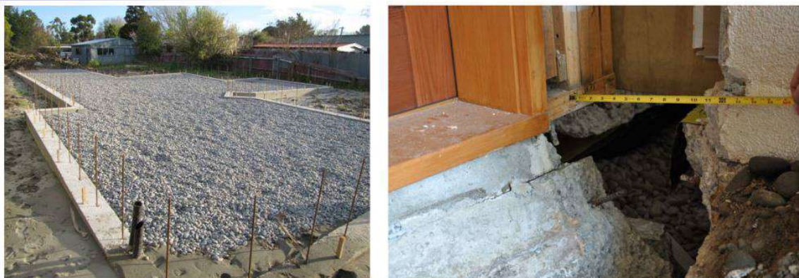
11. Site at Pines Beach which appears to be using the same slab-on-grade system
